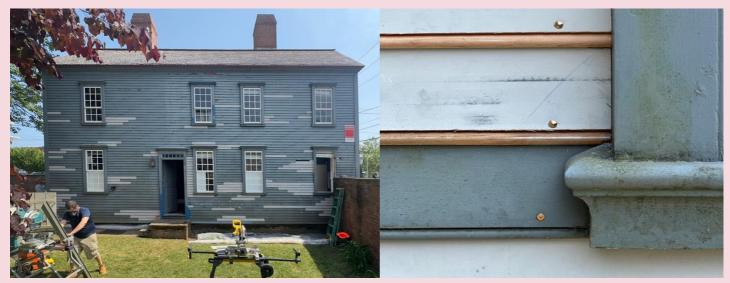
The exterior cladding of **2 Marlborough Street** has been inspected and any siding that has decayed is replaced with freshly milled clapboard. In this case, brass nails are used to reflect the historic construction of the building. Once painted, these repairs will no longer be discernable.
