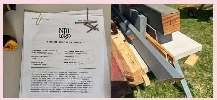
Newport Restoration Foundation has an in-house wood mill. A detailed restoration plan is first created by the Preservation Team (left photo), then each replacement part is milled, labeled, and brought to the site for installation (right photo). Once on site, the milled elements are custom fitted into the existing building envelope. Each of the 70+ houses that NRF stewards has unique millwork needing regular maintenance and restoration.
