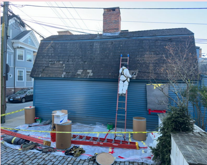
The roof on 181 Spring Street has been completed. The process involved the removal of the previous failing cementitious shingles and foil underlayment, followed by a new water-protection system and wood shingles. The home is now ready for its next tenant-steward to move in.
