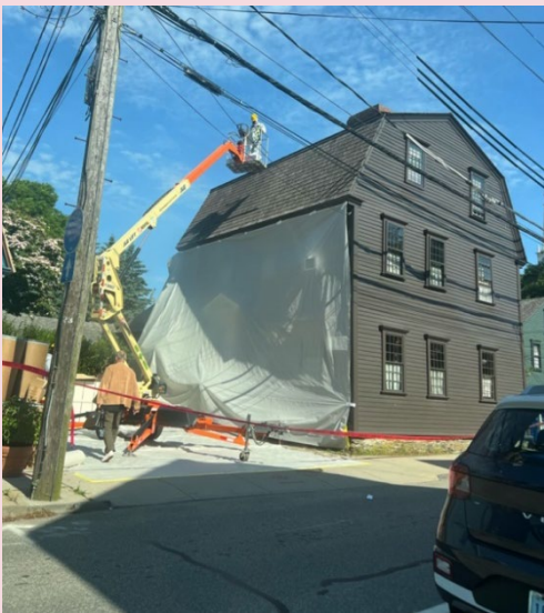
175 Spring Street is sheathed in protective plastic as the work to remove the existing roof material begins. Because of the gambrel roof structure, a hydraulic lift is required. The tight urban fabric of Newport makes this type of work difficult because there is limited space for set-up and removal of debris. Many NRF houses are zero-lot line and rest directly against the pedestrian sidewalk.
