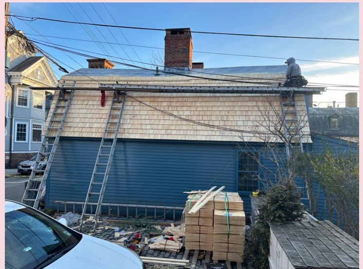
The roof on 181 Spring Street has been completed. The process involved the removal of the previous failing cementitious shingles and foil underlayment, followed by a new water-protection system and wood shingles. The home is now ready for its next tenant-steward to move in.
