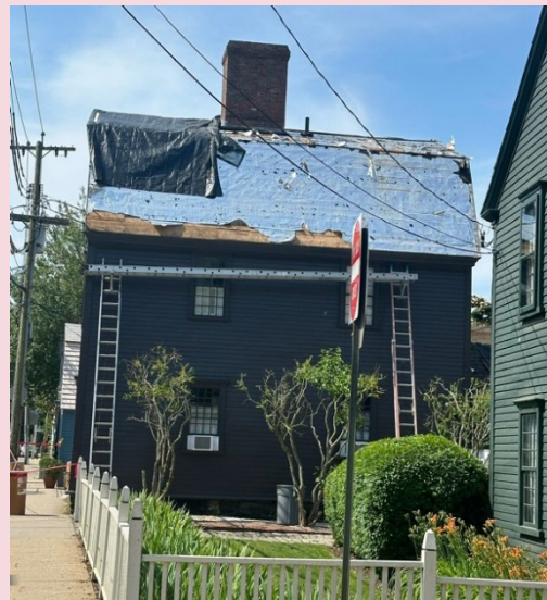
175 Spring Street is sheathed in protective plastic as the work to remove the existing roof material begins. Because of the gambrel roof structure, a hydraulic lift is required. The tight urban fabric of Newport makes this type of work difficult because there is limited space for set-up and removal of debris. Many NRF houses are zero-lot line and rest directly against the pedestrian sidewalk.
